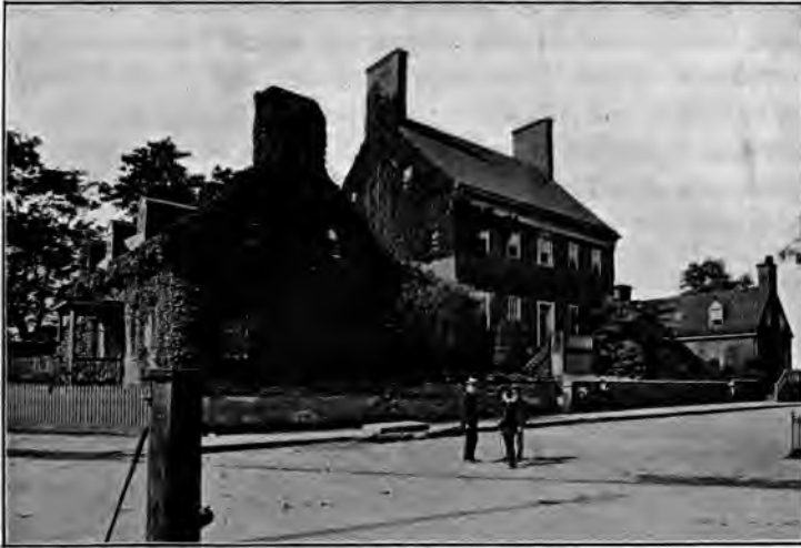
The Brice Residence, Annapolis From a photograph
